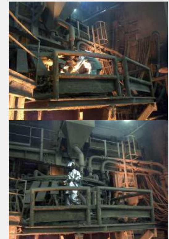
Fig 4 Operator at EBT balcony
